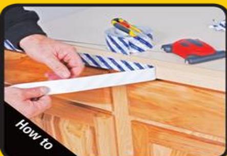
Remove liner, apply edgebanding
