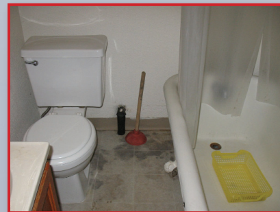
Locate moisture under bathroom floors
