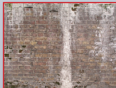
Check for moisture behind masonry
