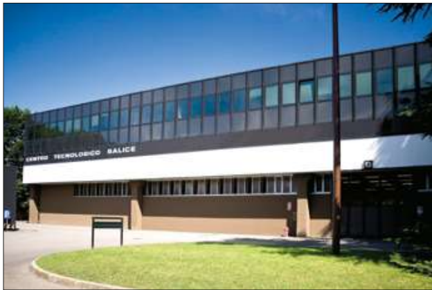
Salice Technological Centre in the Novedrate factory
